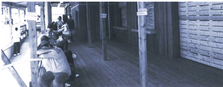
The Rebuild Center, built on the grounds of St. Joseph Church.
