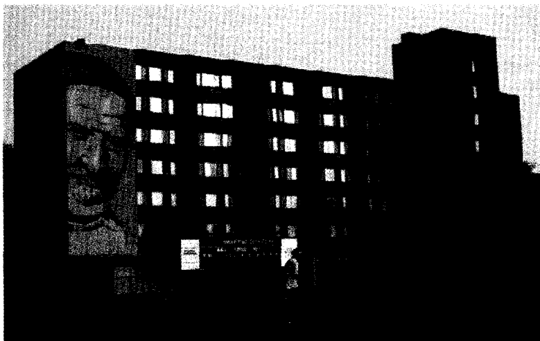
The McCabe Hall Apartments, with mural of Vincent de Paul. DePaul University, Chicago, Illinois. Image collection of DePaul University
