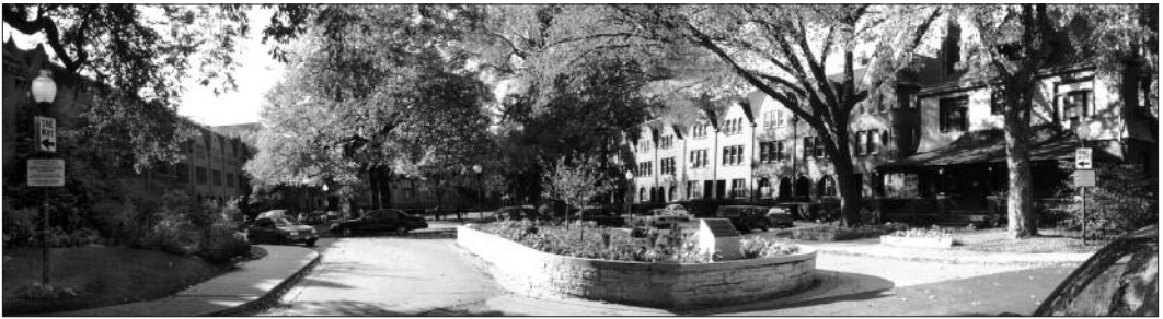
The Chalmers Place Green provides a park-like oasis in the center of the rowhouses, unusual in a dense urban area. The Commons is behind the Green with rowhouses on either side.
